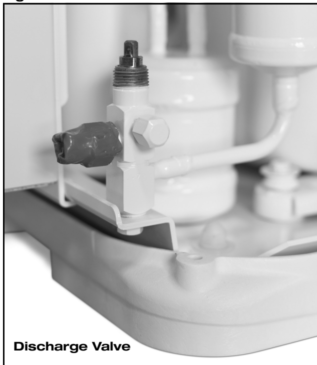
Figure 2: Service Valves Shown in Frontseated Position
