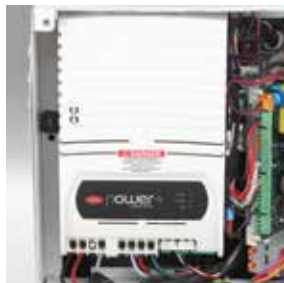
Built-in variable frequency drive.
