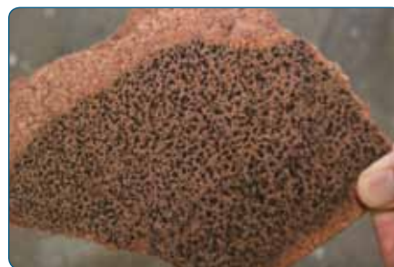
Mold growing on insulation in a yacht
