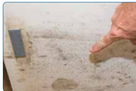
Mold spreading inside a yacht's wall panel
